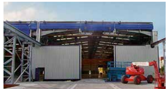
Specialized door designs are possible, such as a T-shape to accommodate a crane on rails.
